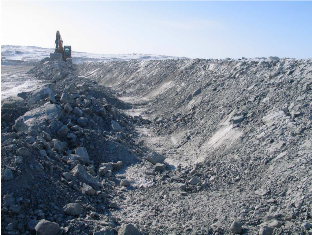
Photo 2: Back sloping down stream berm ~ Sta 2+50 facing west.
