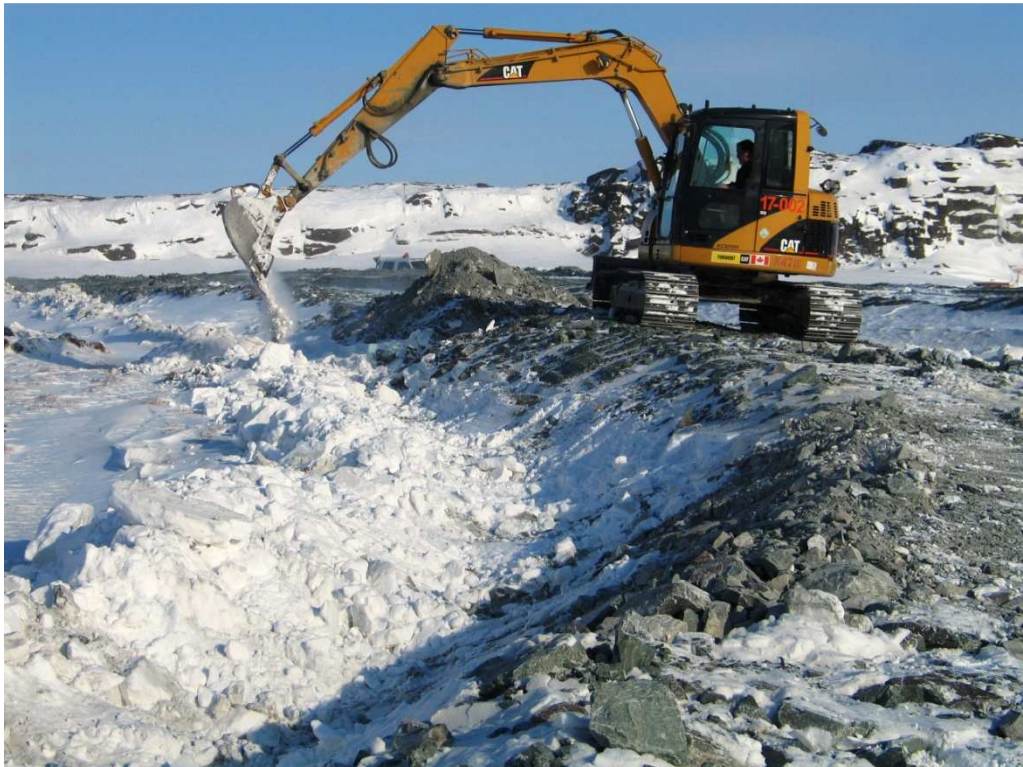
Photo 3: Small excavator trimming up stream ROQ slopes and filling any holes that were left around stakes
