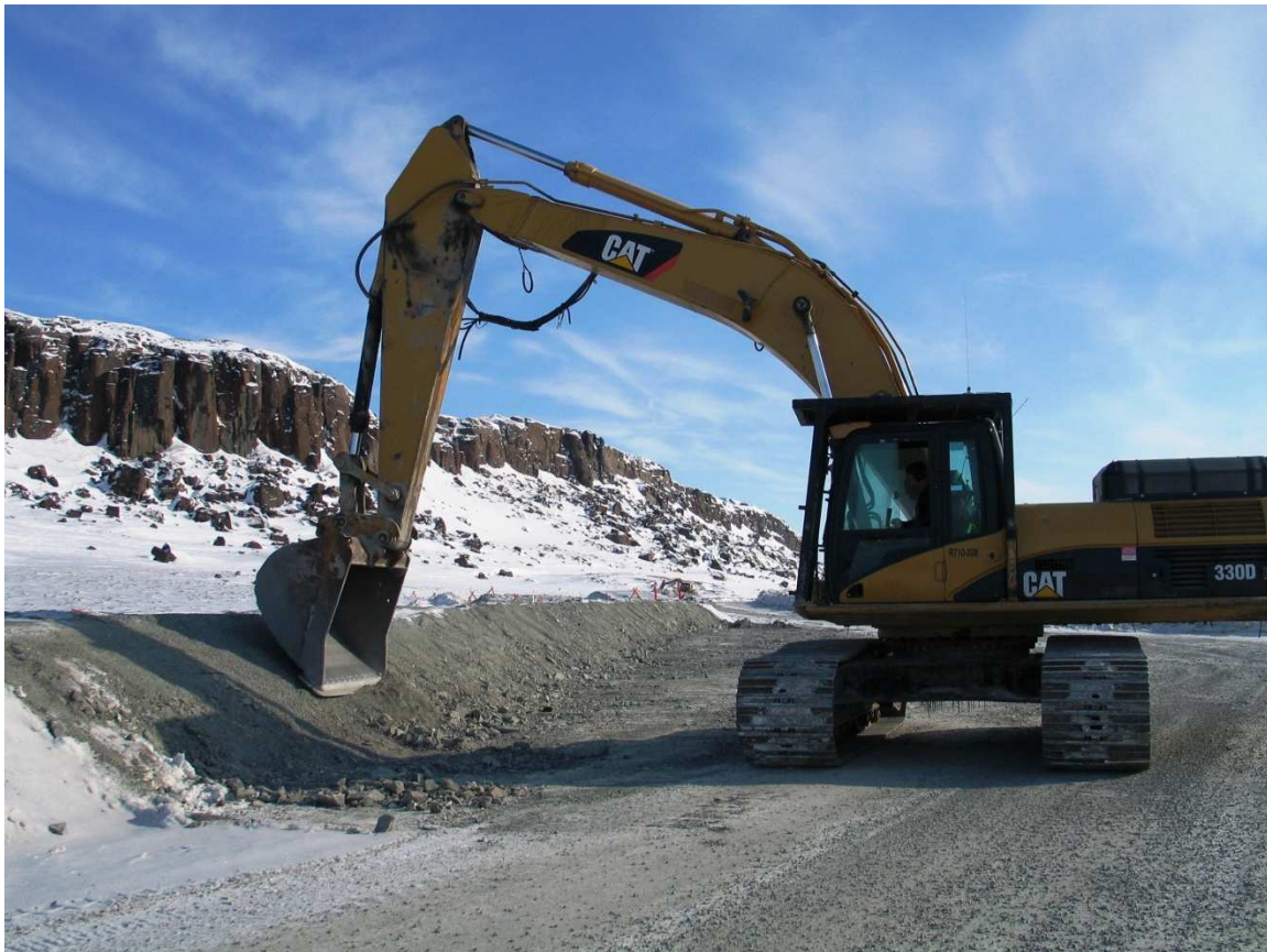
Photo 1: Excavator back sloping downstream berm ~ Sta 1+50 facing east.
