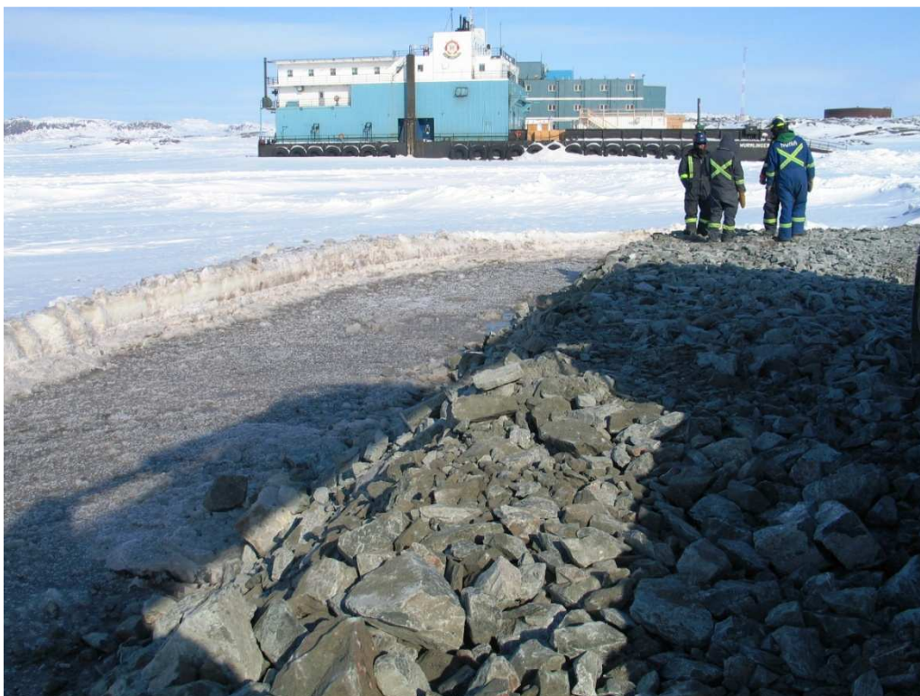
Photo 4: Work at the jetty. Ice removed and excavation complete.
